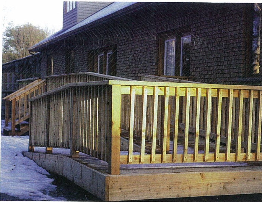
A gently ramped porch makes the backyard easily accessible.
